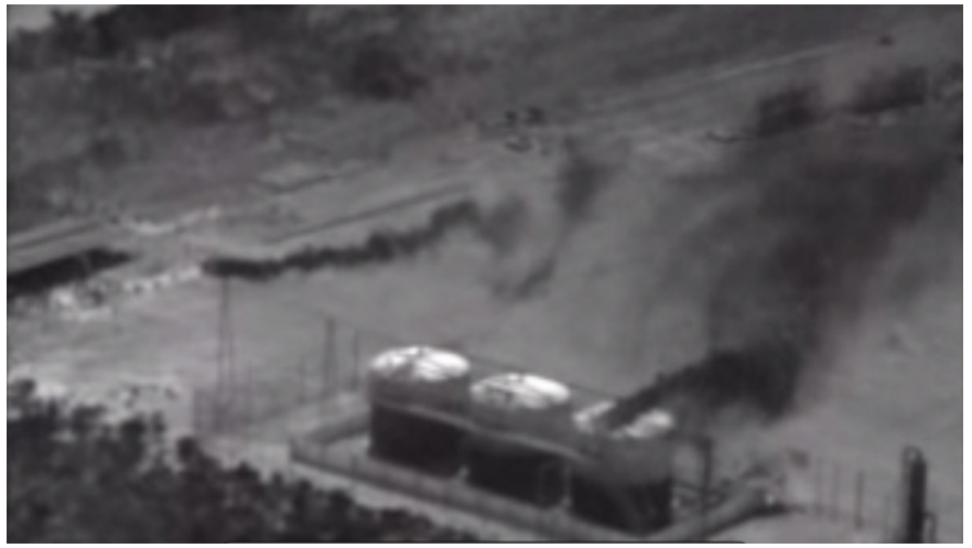
Volatile Organic Compound (VOC) pollution escaping from a gas condensate tank in the Barnett Shale as photographed by a TCEQ infrared camera.
