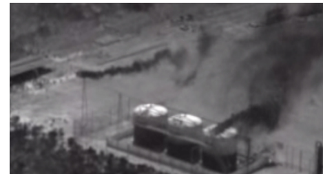
Top: Gas condensate tanks as they appear to the naked eye. Bottom: Those same tanks as they appear to an infrared camera. Those are plumes of VOCs being released.
